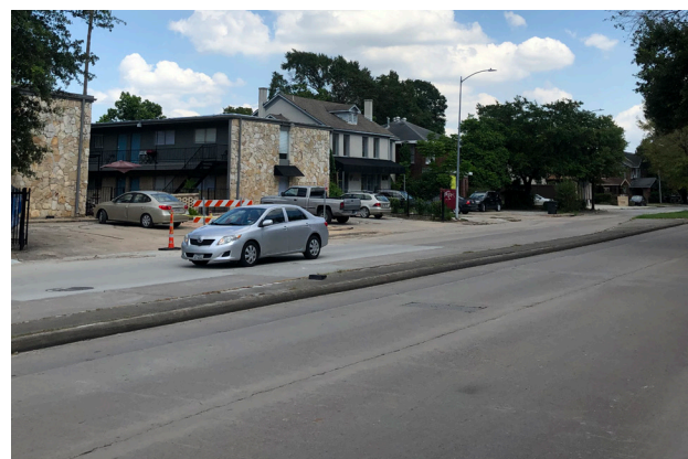
Richmond Avenue is a narrow right-of-way where a more narrow pedestrian realm requirement may be established.
