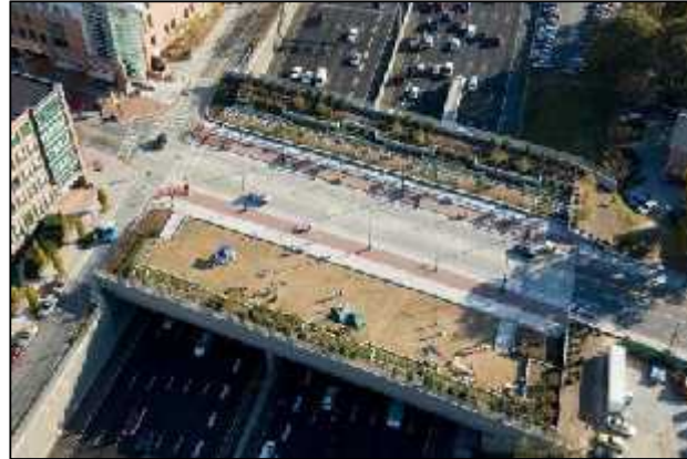
5th Street Bridge Atlanta
