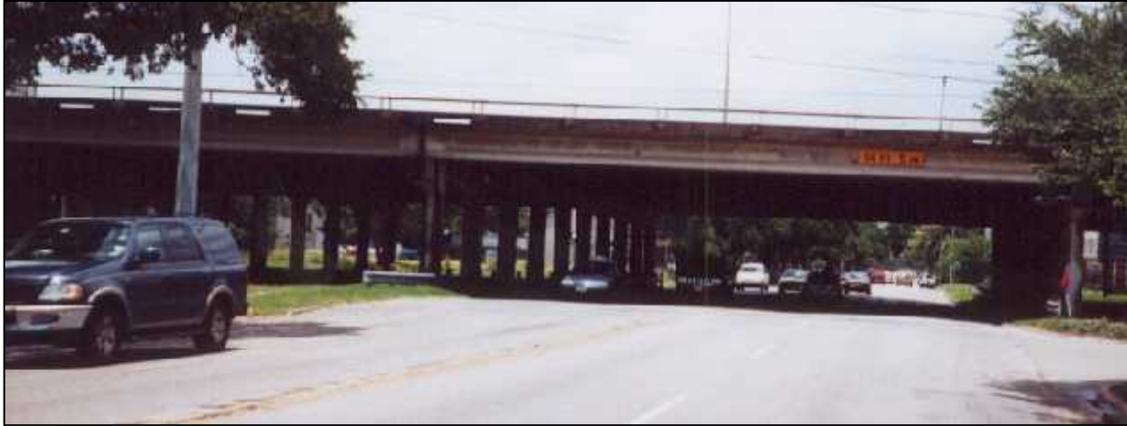
Montrose Underpass - Before
