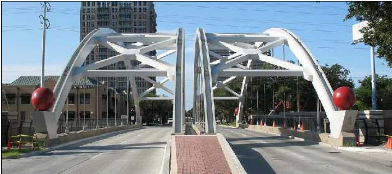
Montrose Bridge - After
